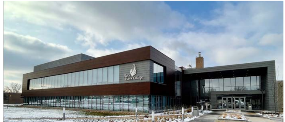
Building 1 - Addition & Renovation
